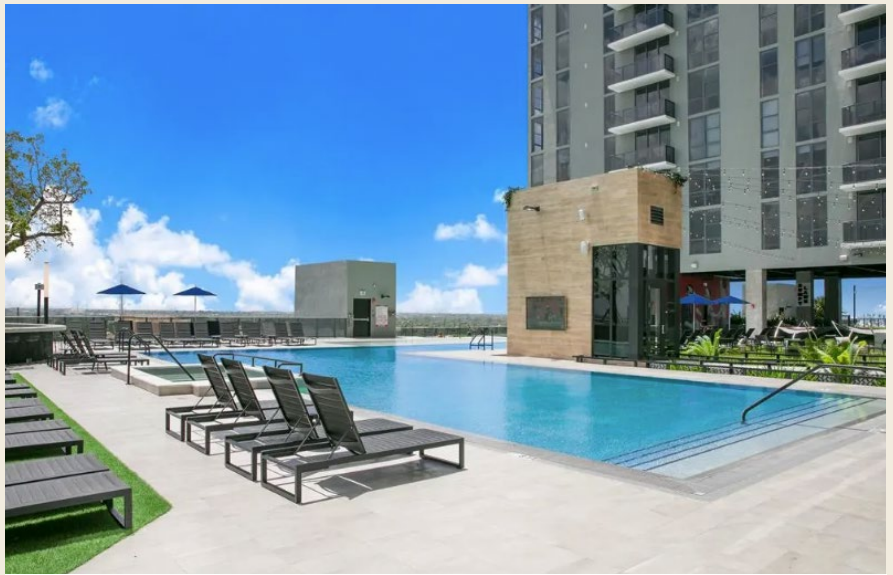
RESORT STYLE ROOF-TOP POOL DECK
