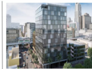
NIKOLA TESLA INNOVATION HUB 155 S Miami Avenue Downtown Mixed-Use with 137,000 SF Class A Office Space & 6,000 SF Retail Space Typical Office Floor: 10,461 SF Delivering: 3Q 2022
