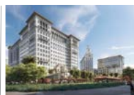
THE PLAZA CORAL GABLES 2811 Ponce De Leon Blvd. Coral Gables South Tower 163,700 SF Typical Office Floor: 22,744 SF Delivering: 4Q 2021
