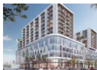
STRATA 2221 N Miami Avenue Wynwood Mixed-Use Project with 60,300 SF of Class A Office Space, 27,210 SF of Retail Space, and 257 Residential Units Typical Office Floor: 20,100 SF Delivering: 4Q 2021
